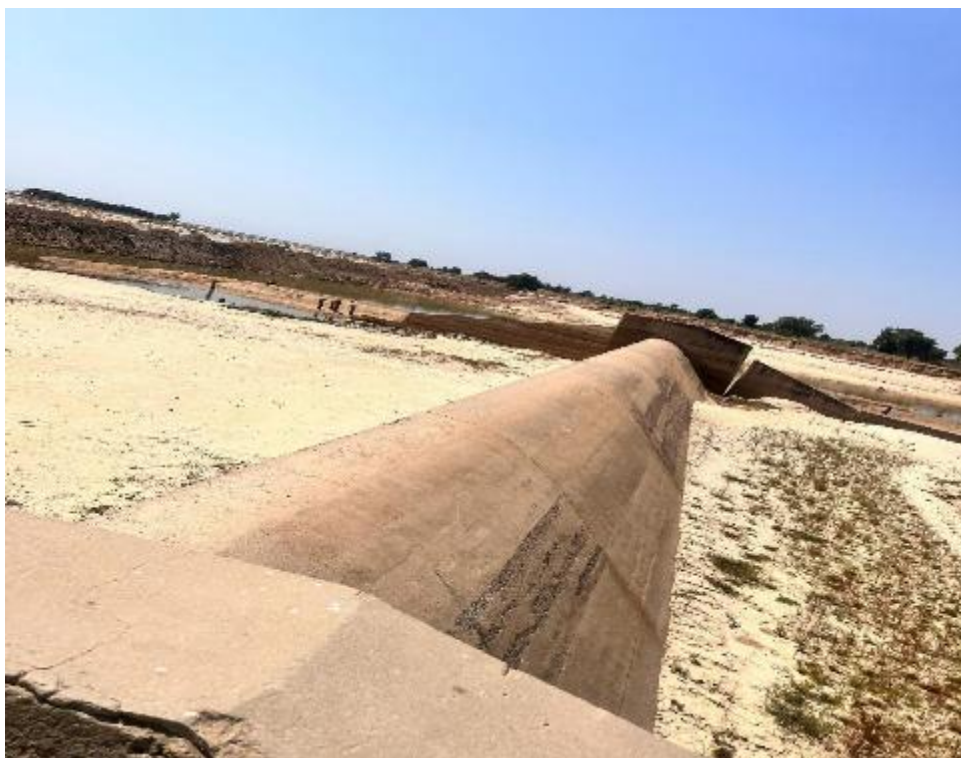
Figure 4: Collapsed Dyke
