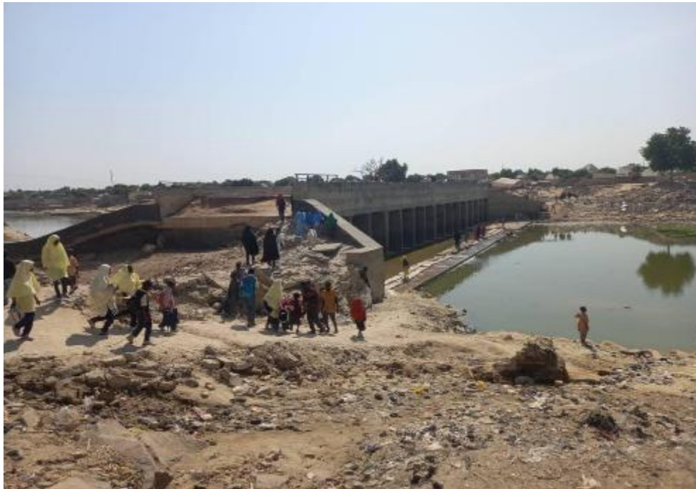
Figure 5: Collapsed Fori Bridge
